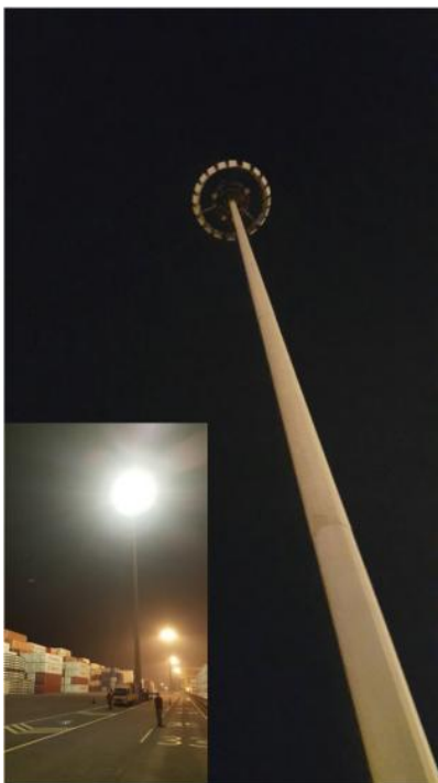
Pole light in Airport / Dock / Logistics Center
